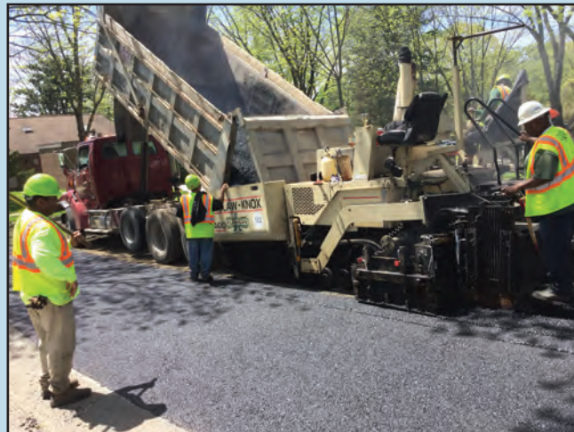
Aging Infrastructure Maintenance
